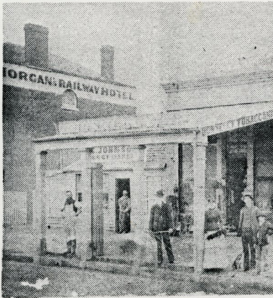
ABOVE: Northern aspect of the Railway Hotel.
